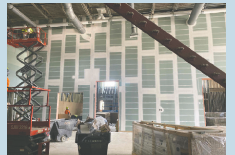
Drywall going up in the main lobby facing the new auditorium/multipurpose space
