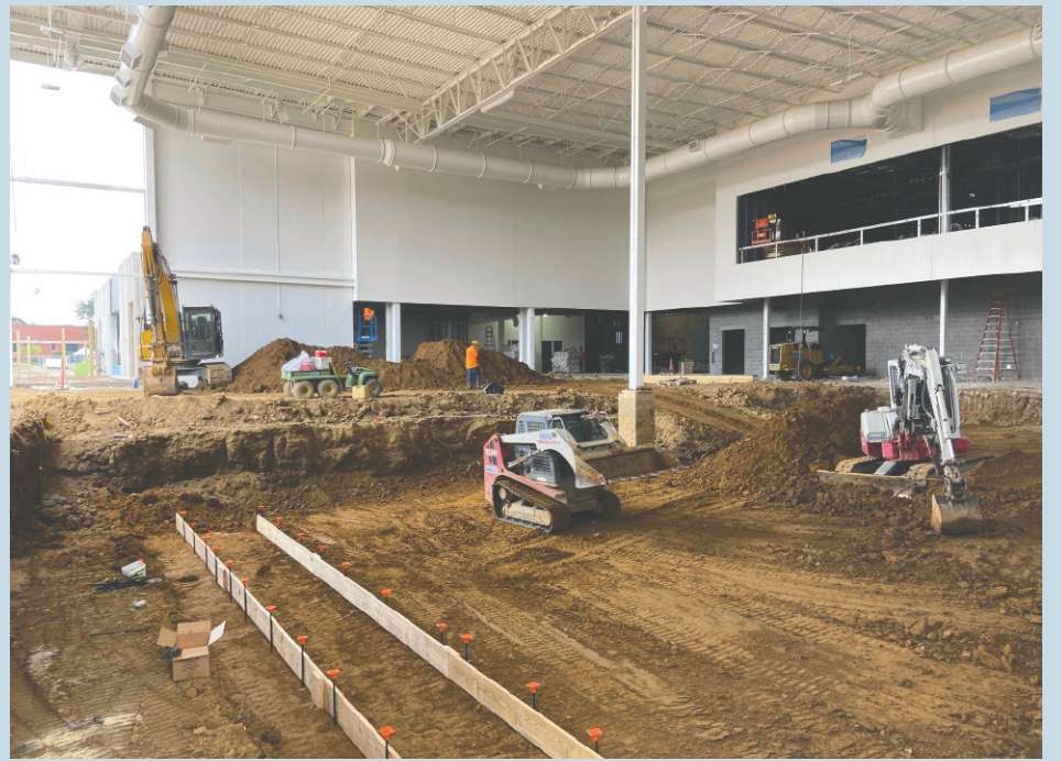
Indoor family pool area being dug with heavy digging equipment
