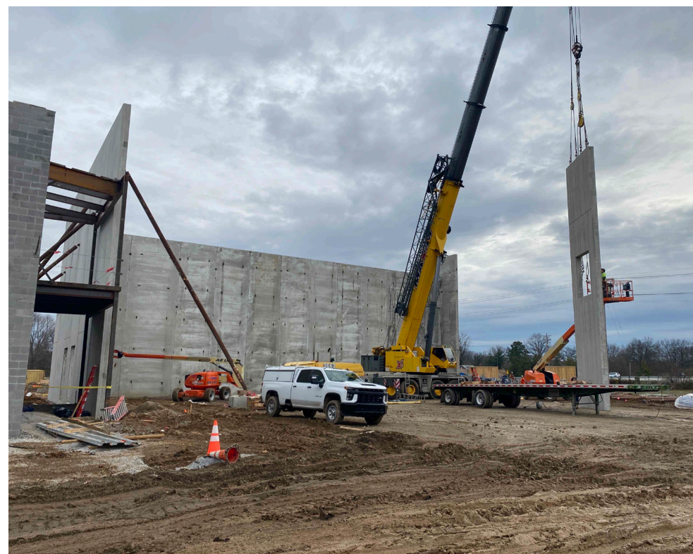
Construction continues on the future Jewish Community Center. Work on the concrete exterior panels and steel is nearing completion. The outline/curbing for the new parking lot and driveways is well advanced. The elevator shaft is in and roofing will soon be installed. (JCC photo)
