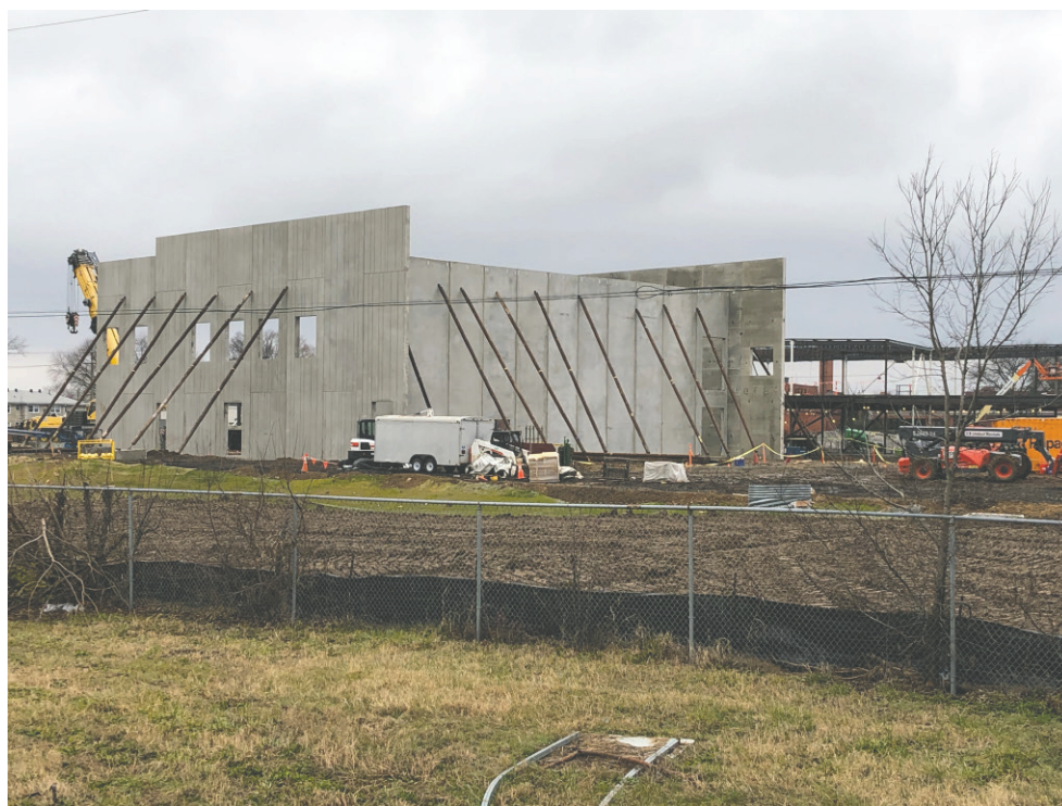
The walls of the future Jewish Community Center of Louisville are now being erected. The pre-cast concrete panels, which will form the exterior walls of the JCC, will allow placement for windows and doors without further modification. Most of the walls already up encompass what will be the exercise area. Work on this aspect of construction is expected to be complete by mid-February. (Community photo by Lee Chottiner)
